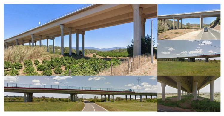
Detailed design of 11 viaducts, 30 overpasses or underpasses and a cut-and-cover tunnel. The deck typology of the viaducts includes 2 precast concrete U-beams, which are subsequently continued by means of post-tensioning with high yield bars. The viaducts have dampers in the abutments to dissipate seismic forces.
